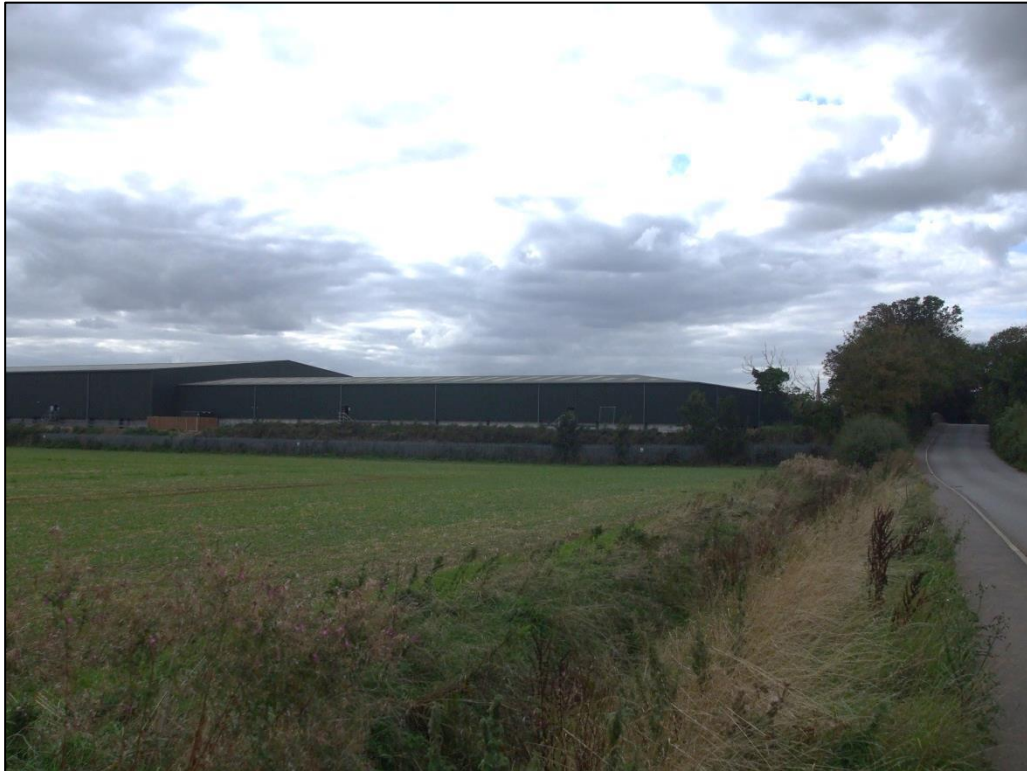
View of site from the east, Caythorpe Heath Lane
